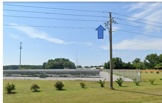
Point of Common Coupling (PCC)
