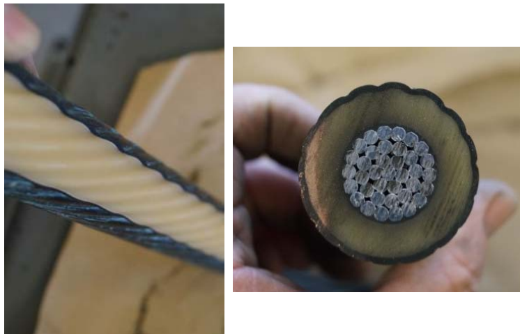
Figure 5: Cable Deformation Due to Elevated Temperature Operation
